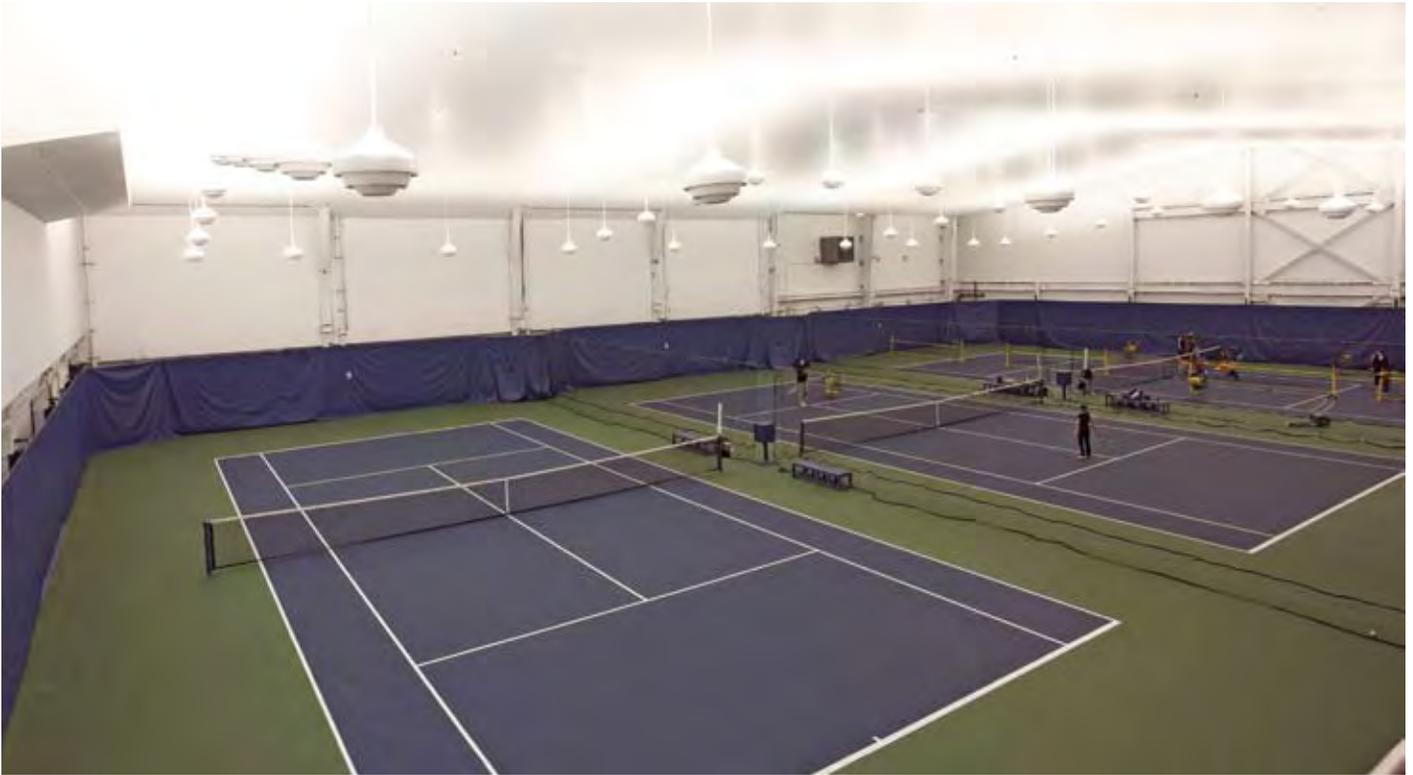
***The column-free space for the interior courts required 120-foot clearspans, and the courts had different load requirements than other areas of the building, making the initial planning process challenging.***
