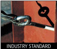
No matter how strong the building, the bracing system is its backbone. Over the years, Butler steel-rod bracing retains its original strength and tightness. It doesn't stretch or sag like wire rope and cable, allowing your building to move or rock under wind loads.
